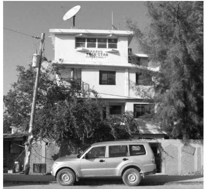
Pastor Benoit's 4 story church building. The sanctuary at the bottom floor is woefully too small, they spill out into the courtyard at every service.
